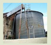
A tank made from corrugated iron.<sup>2</sup>
