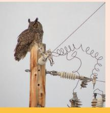
The pole is made of wood which does not conduct electricity and there are ceramic caps between the power lines and the pole which act as further insulators.
