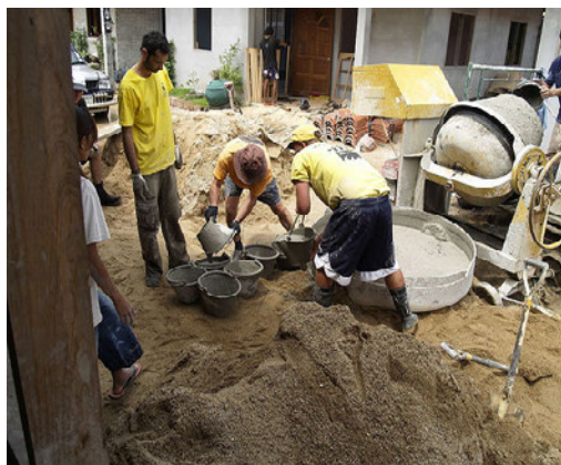
Mixing cement using a mixer.
