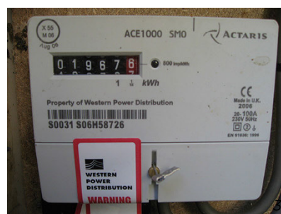
An electricity meter. Can you see the number recording the electricity usage in kilowatt hours (kWh)?
