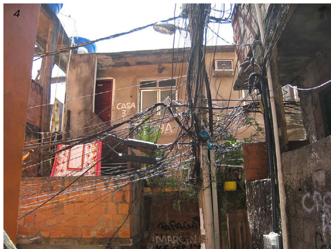
Look at this mess of illegal electrical connections.
